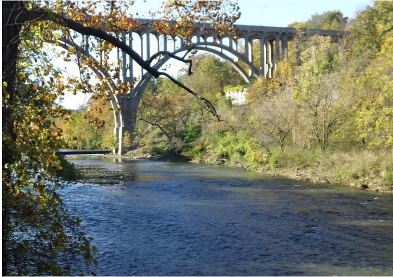
27a. Middle river area near St Rt 82 dam.
