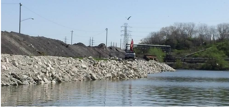
27c. Rip rap area at Arcelor Mittal.
