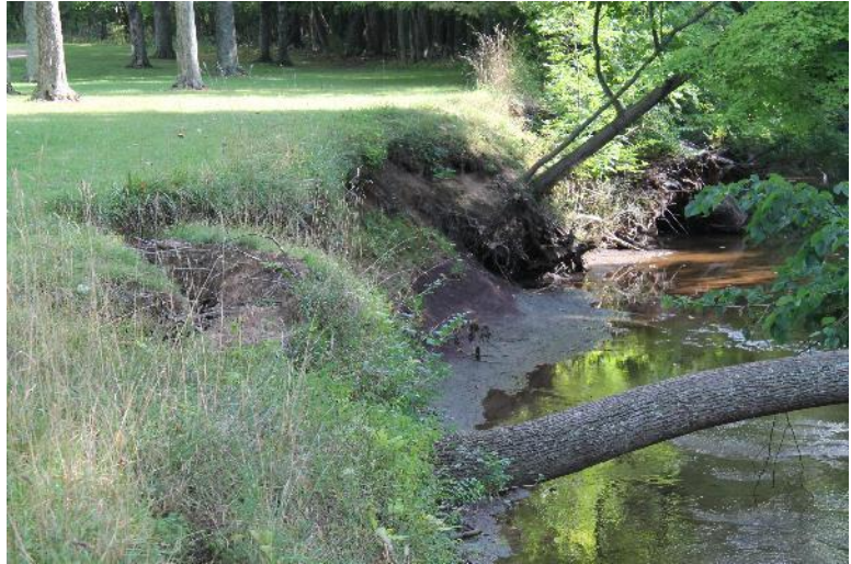
Figure 2. Eroding banks along Big Creek.
