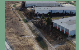
West Creek Flume Fish Barrier Removal
