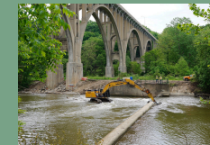
Canal Diversion Dam Removal
